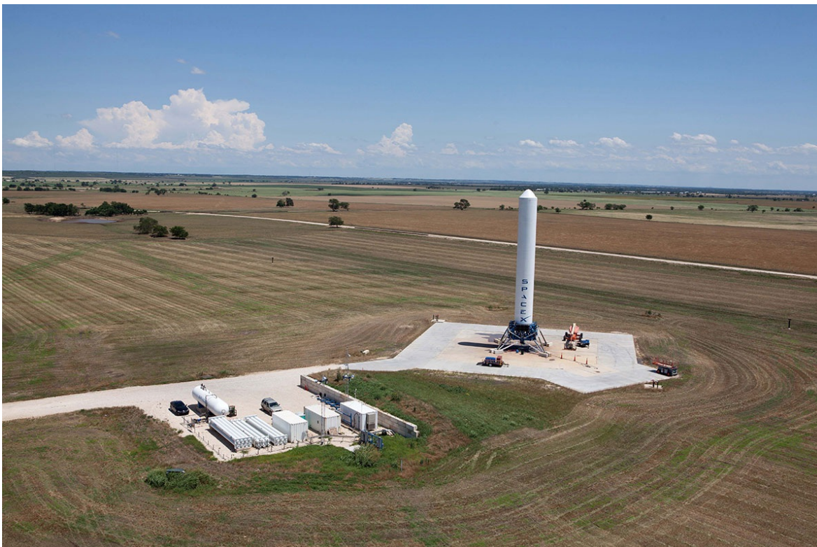
The SpaceX facility in McGregor, Texas.
